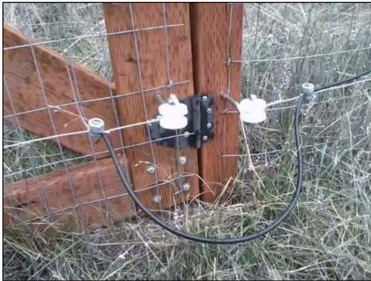
*Figure 5. Black-colored insulated electric fence wire, 12-gauge. Used here to connect the electrified lines of a gate to the main electrified lines on the fence.*
